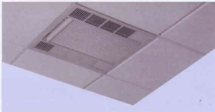
The X-400 features the 'Coanda' 4-way airflow pattern.
